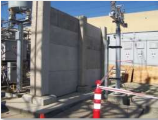
Physical Firewall at Electrical Substation
