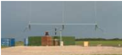
Figure 25: Anthorn eLoran Transmitter
