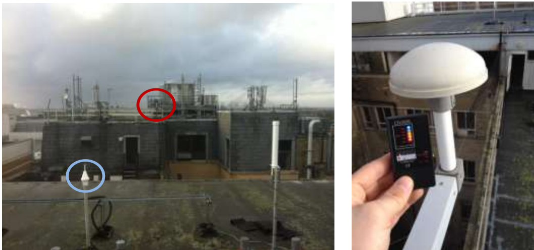
Figure 20: Rooftop location of reradiating (red) and victim (blue) antenna.
